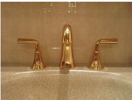
Sink in toilet room
