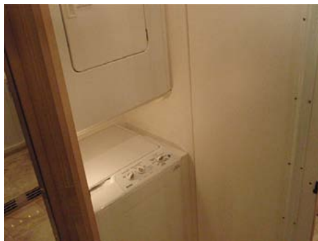
Concealed stacking washer and dryer
